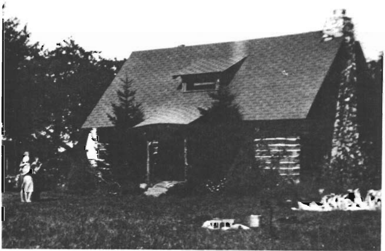
DENOYER LOG CABIN was the local campsite for Wheeling Girl Scouts for many years. It had tables, chairs and a piano on the ground floor and a loft where the campers slept.
